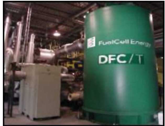
Fig. 11. FuelCell Energy's DFC/Turbine hybrid system.
